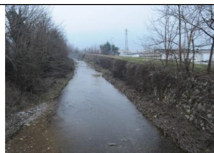
Bank walls with the function of levees
