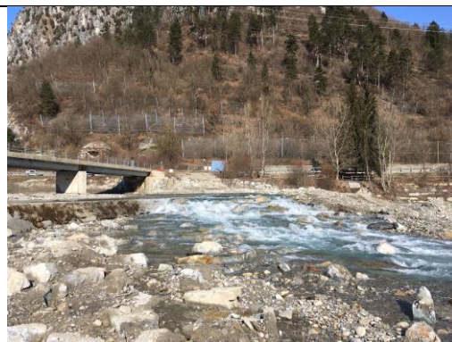
Ramp below a sill to facilitate fish passage
