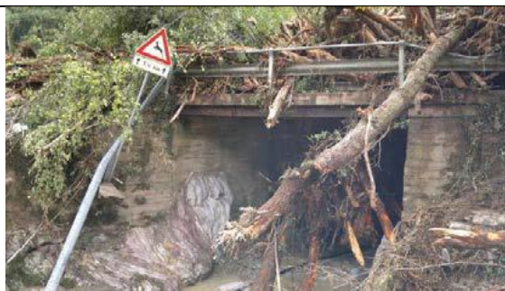
High single arch bridge but with a small width, not enough to allow intense transport of large woods
