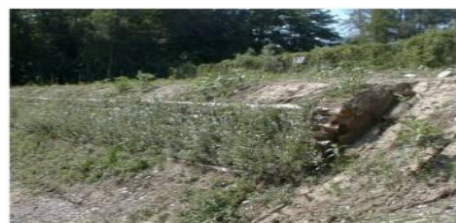
Bioengineering bank stabilisation
