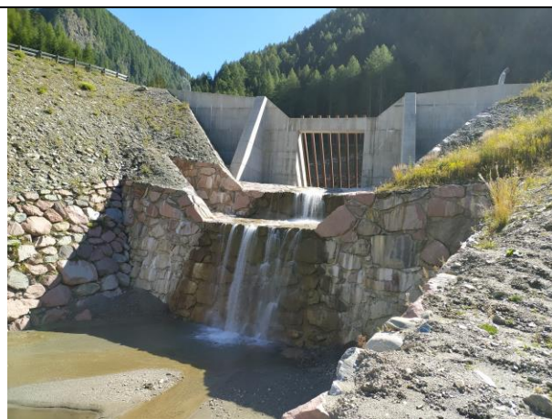
Selective retention weir associated to two consolidation weirs downstream
