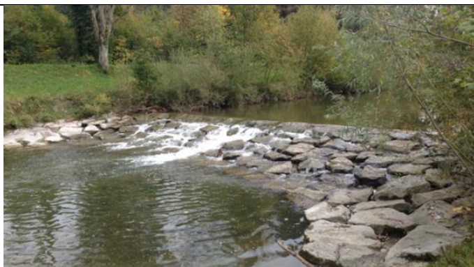
Ramp with boulders
