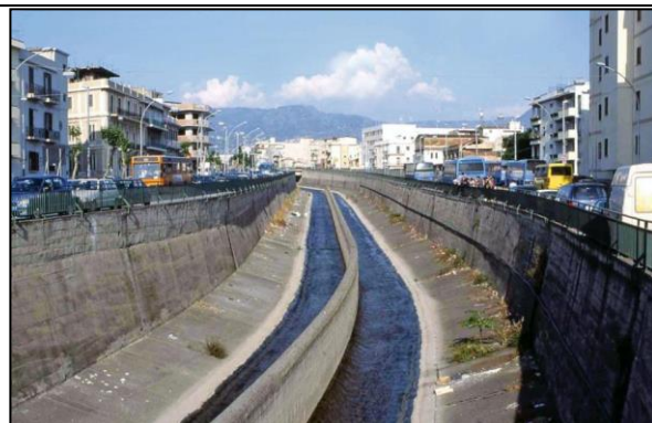
Concrete bed revetment in stone (left) and concrete (right)
