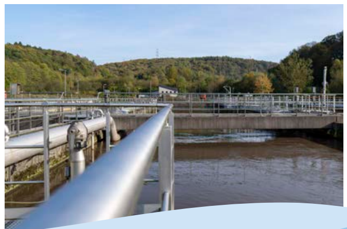
Kohlfurth treatment plant
